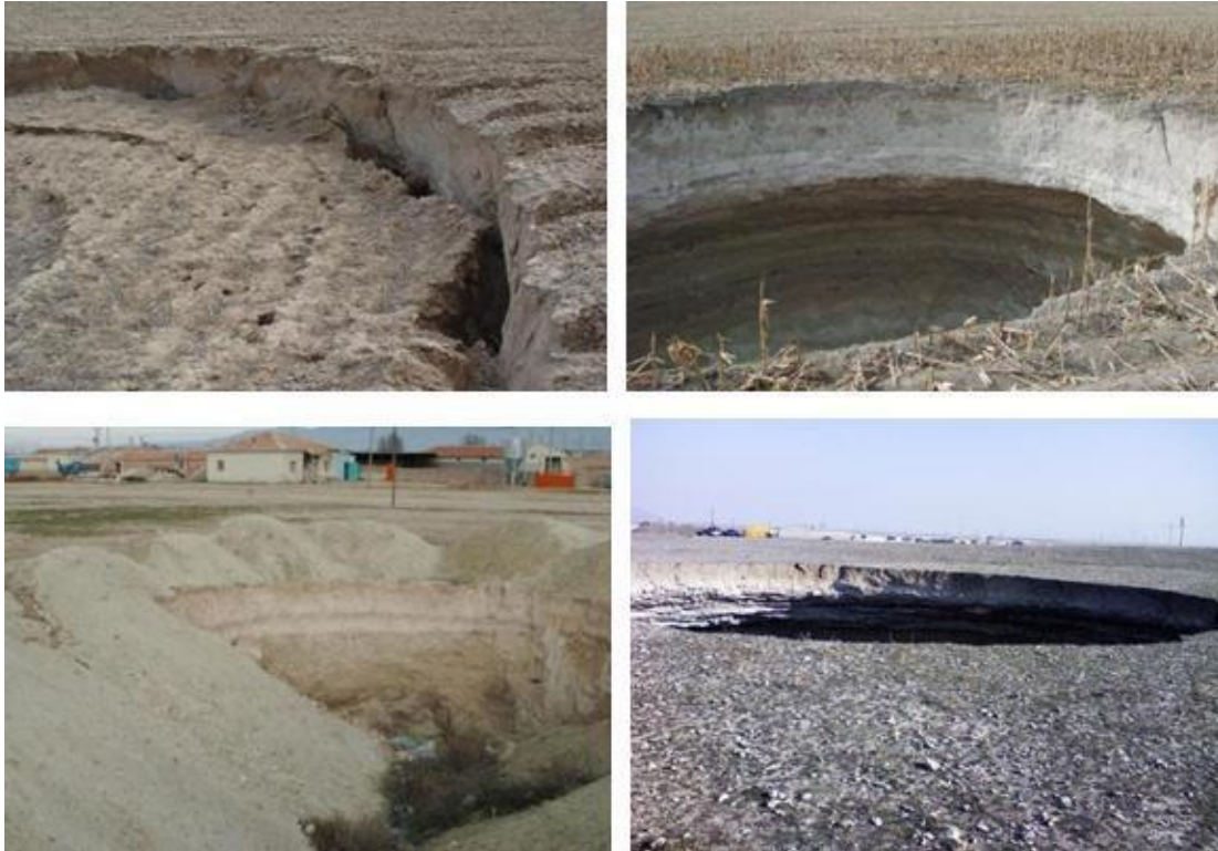
Figure 1. Agricultural sinkholes from central Turkey.
