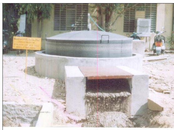
Figure 4. Jatropha based biogas plant (floating drum type).
